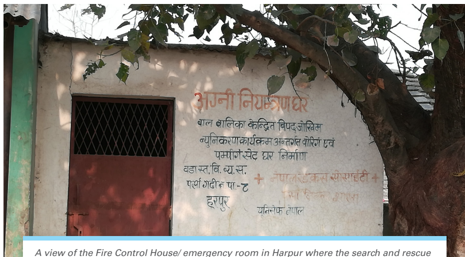
A view of the Fire Control House/ emergency room in Harpur where the search and rescue equipment and water pump are installed.
